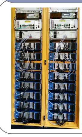
The laboratory has a number of test stands available for the development of advanced diagnostics, ultra-fast syncrhonisation systems, electronic processor boards, control hardware and fast digital feed-back systems. The photo on the left shows an equipment rack built for tests in series of button beam position monitors, built at PSI as part of Switzerland's in-kind contribution to the European X-FEL project.
